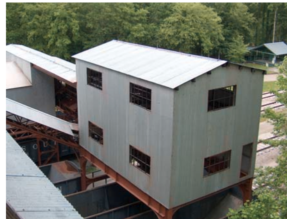
Top left: A reconstructed tippie and bridge sits at Blue Heron mining camp at Big South Fork (photo by Bill Gee). Top right: These stairs lead up the bluff at Blue Heron (photo by Bill Gee). Left: Wild flowers frequently encroach on the trail at Big South Fork (photo by Bill Gee). Above: The tippie building at Blue Heron (photo by Bill Gee).
